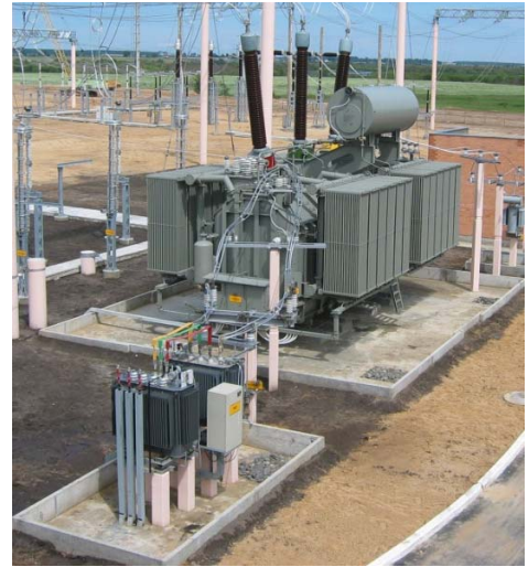
MCR 180 Mvar, 330 kV, Belarus
